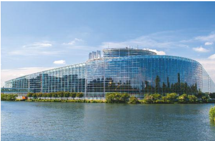
Building automation with Oventrop components and systems: European Parliament in Strasbourg, France
